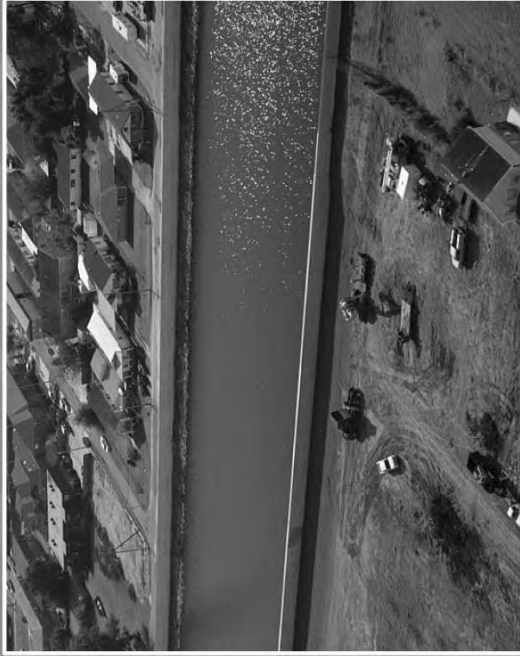
Reconstructed Levees, New Orleans, Louisiana
